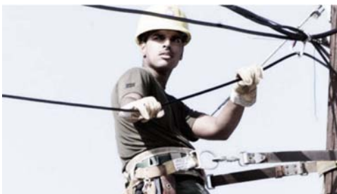
Figure A-20 Line Technician
